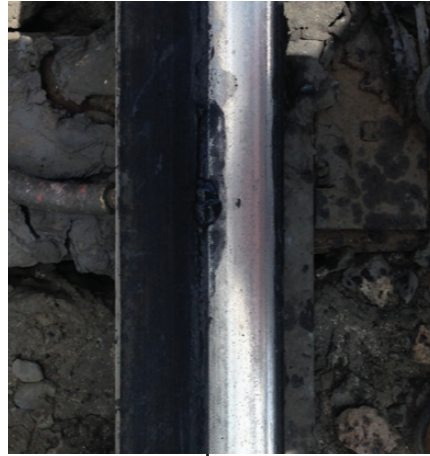
TOR Armor filling holes in rail head.
