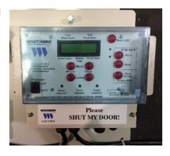
The first wheel of the train initiates the pump. The control panel counts the set number of wheels and then operates the pump grease / friction modifier is then dispensed every time the set number of wheels has been detected.
