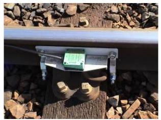
• Adjust the height of the sensor to 42 / 45mm below the rail head crown and securely tighten the M16 fixings.
